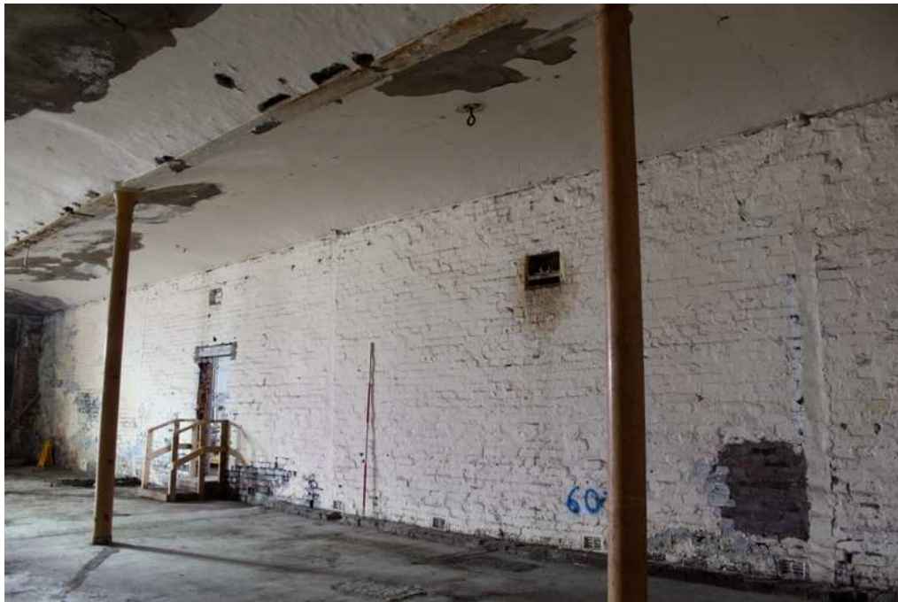
Plate 58: Columns incorporated within inserted brick partition in the weaving shed
