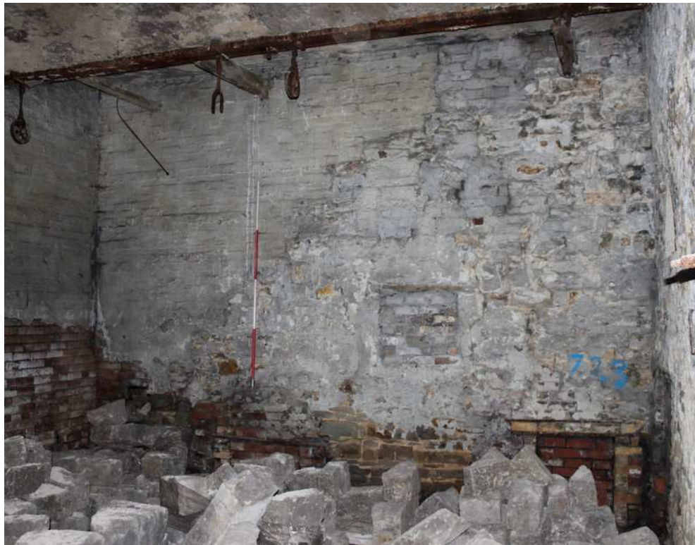
Plate 53: Blocked, refractory brick-lined flue in south east wall of boiler house, with pulley wheels for dampers on the ceiling beams above
