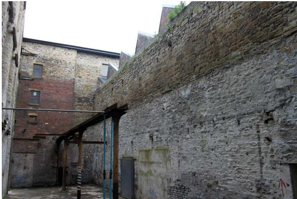
Plate 7: Interior of original spinning block, with inserted columns carrying the valley of a double-span roof
