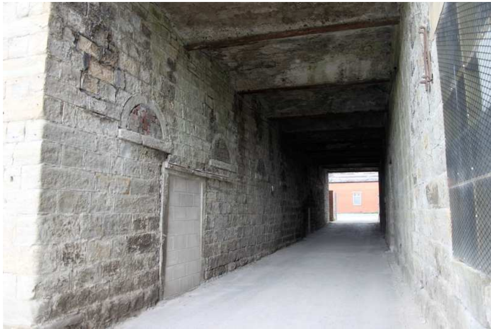
Plate 49: Passageway with apertures into earlier structure and fireproof vaulted ceiling below first-floor weaving shed
