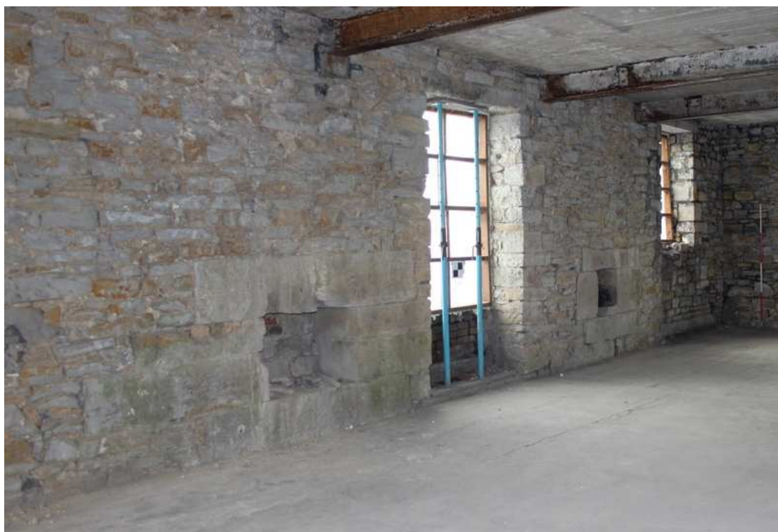
Plate 13: Large apertures associated with the engine, with dressed sandstone surrounds
