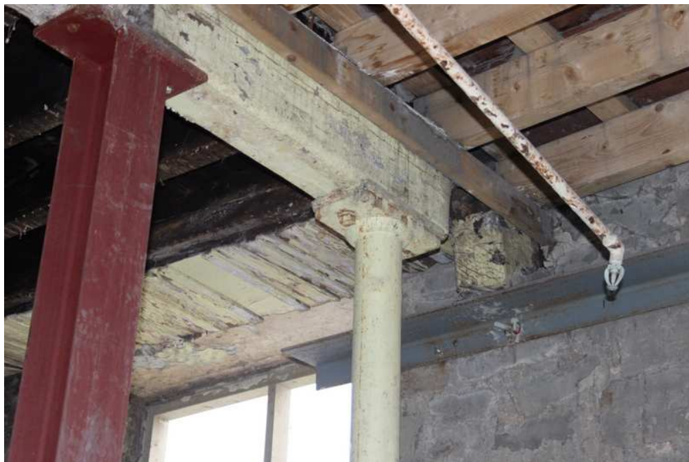
Plate 27: Additional column inserted at first-floor level to carry cut ceiling beam
