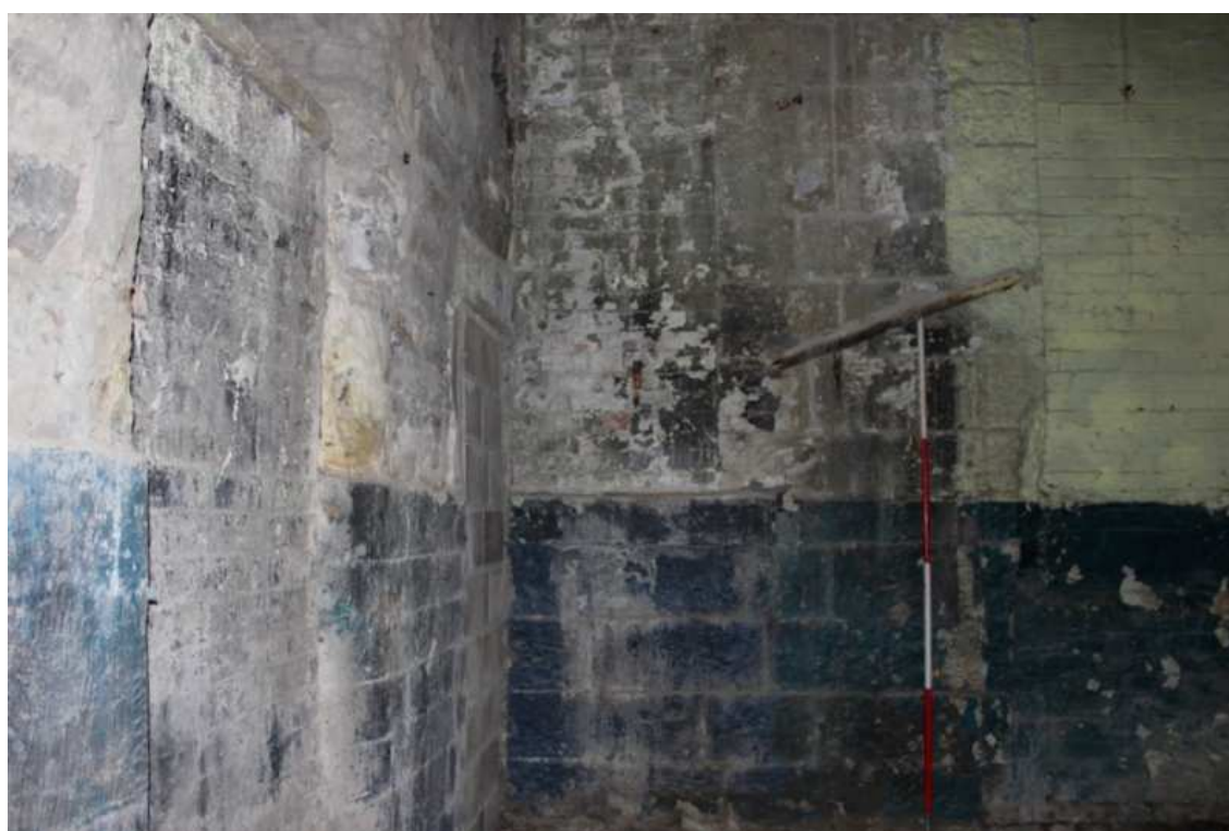
Plate 18: Detail of the south-east corner of the ground floor, with original projecting sill of the earlier spinning block
