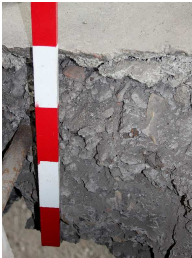
Plate 50: Detail of concrete ceiling arch construction
