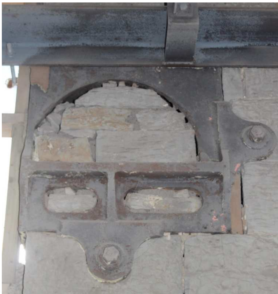
Plate 30: Ornate end bearing box at first floor level
