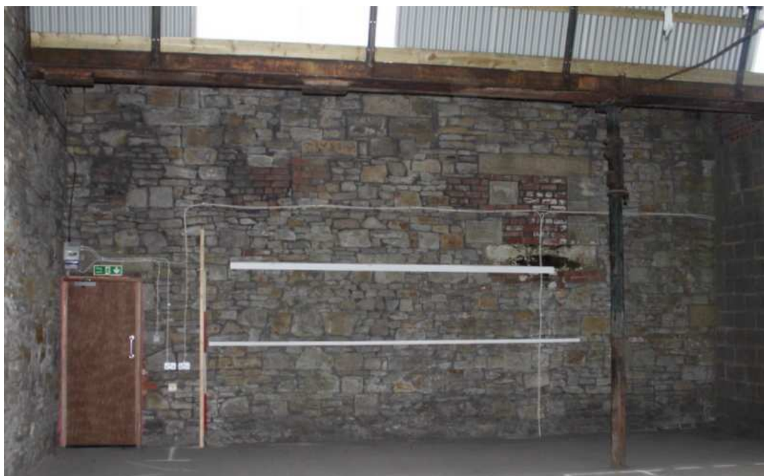
Plate 70: Columns incorporated within inserted brick partition in the weaving shed
