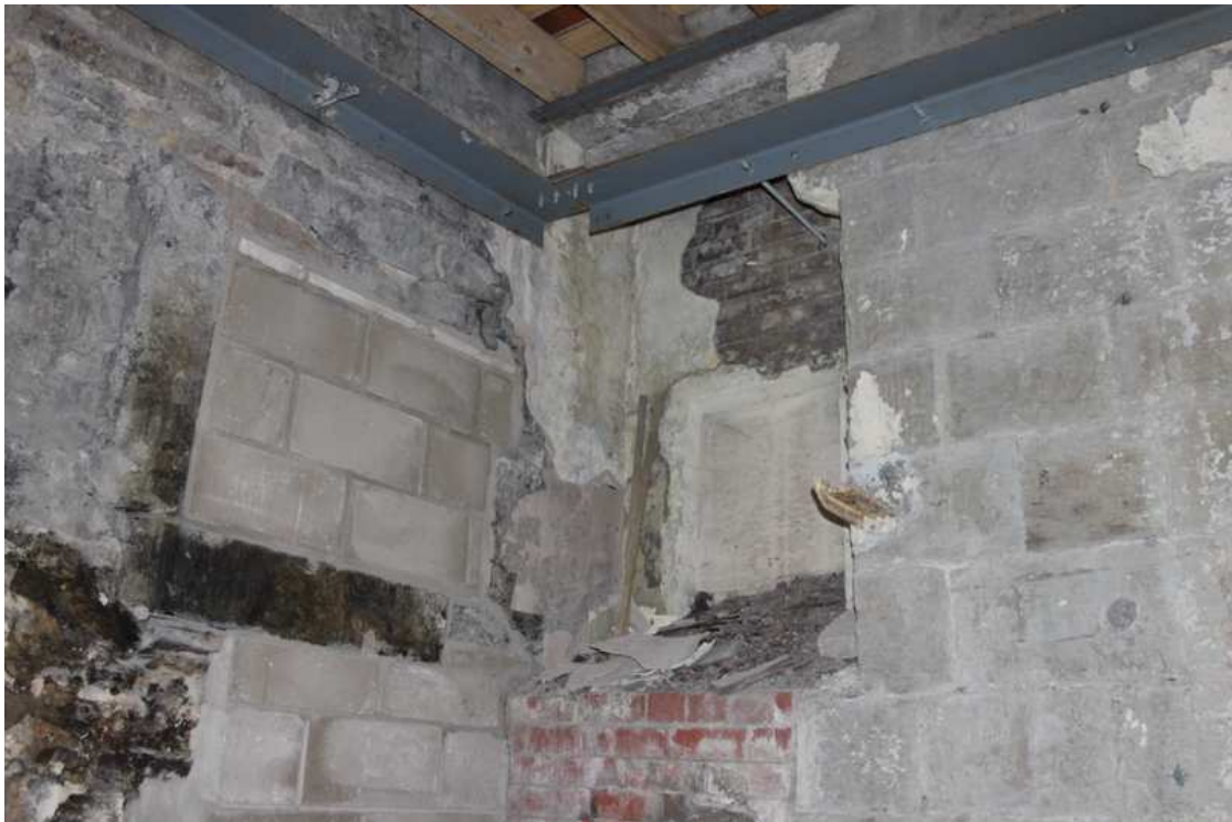
Plate 29: Bearing boxes in south-east corner of first floor
