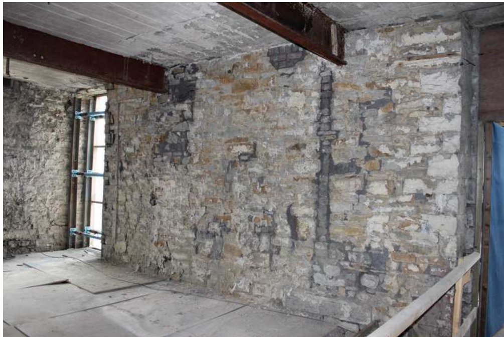
Plate 10: Blocked and inserted apertures in the north-east wall of the engine house, first floor
