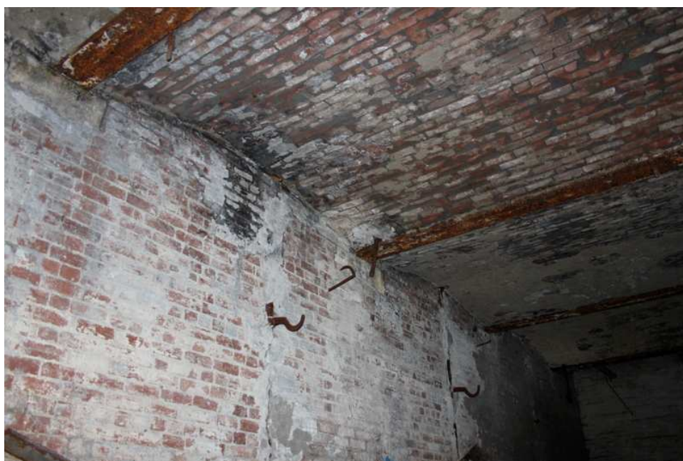
Plate 55: Earlier columns concealed within brick partition, with brick vaulting above
