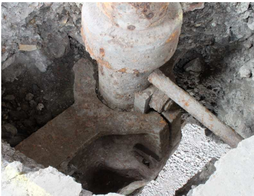
Plate 51: Detail of column jointing between floors of the weaving shed
