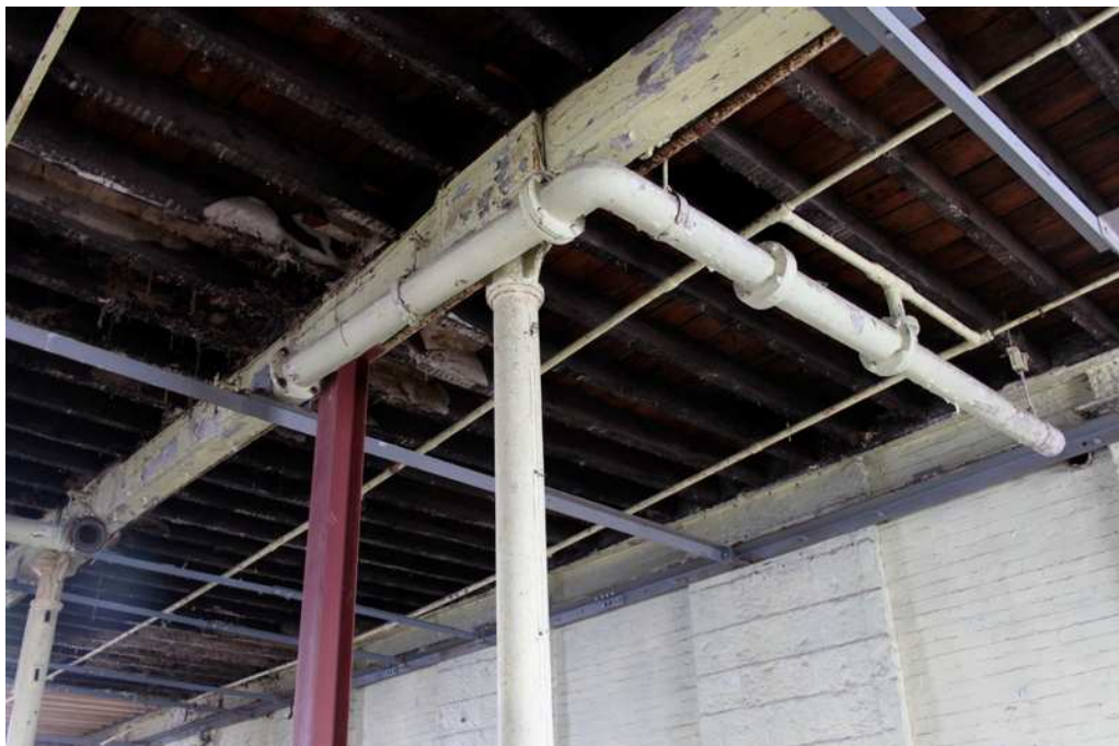
Plate 23: Main sprinkler pipe at ground floor level
