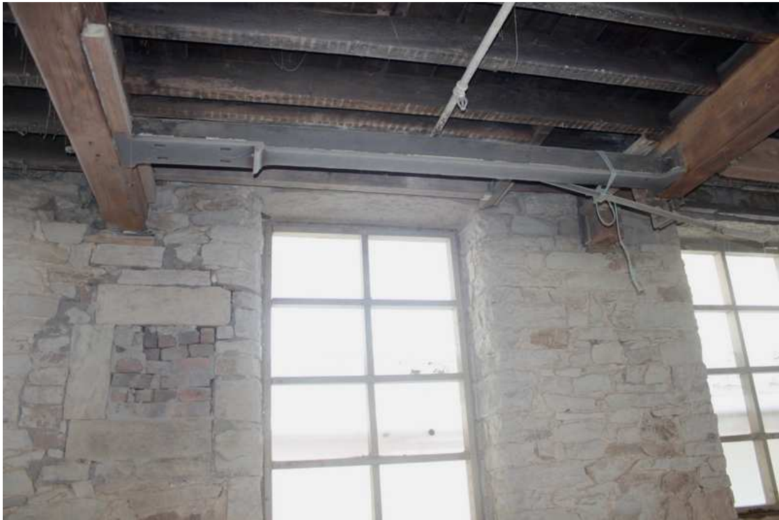
Plate 31: Cast-iron beam with bolting plate for line shaft hanger above blocked end bearing box in wall
