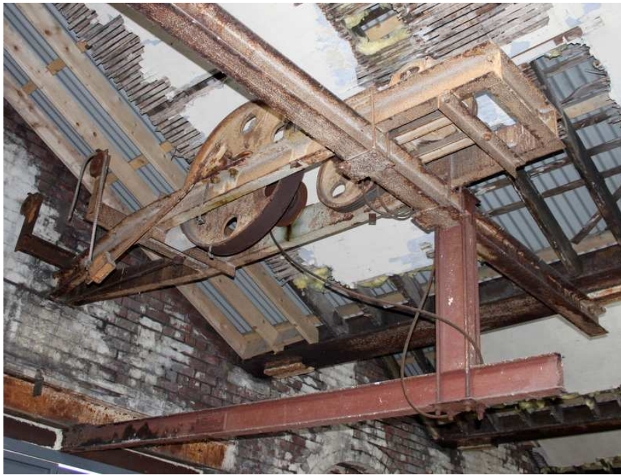
Plate 64: Inserted hoist, attached to line shaft hanger bolting plate
