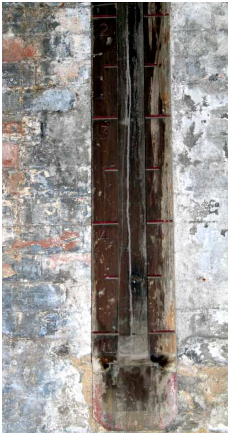
Plate 47: Water level gauge for sprinkler system header tank
