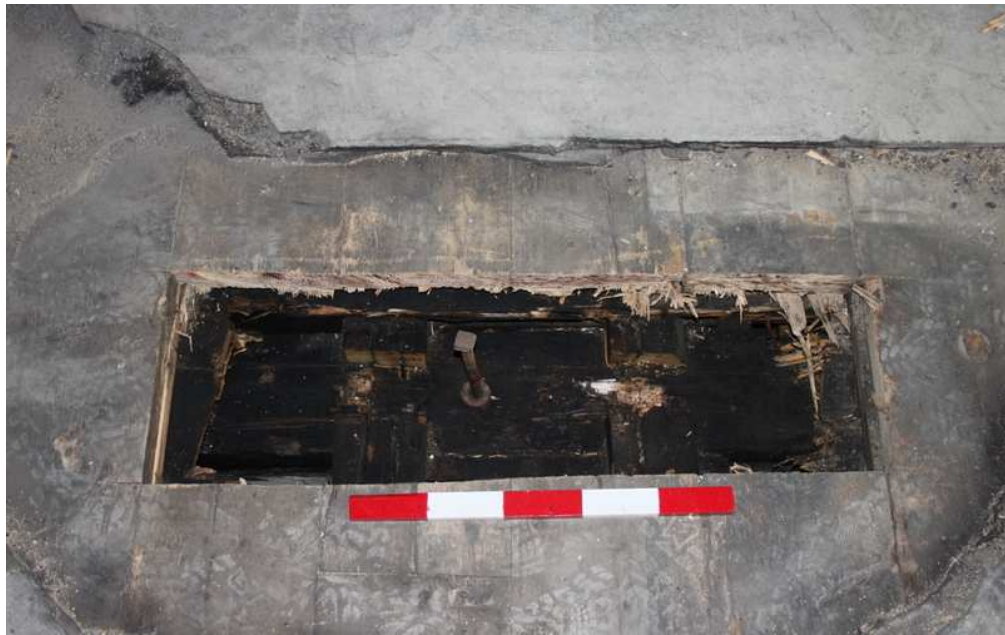
Plate 26: Detail of crush box of ground-floor column and jointing to original position of column above
