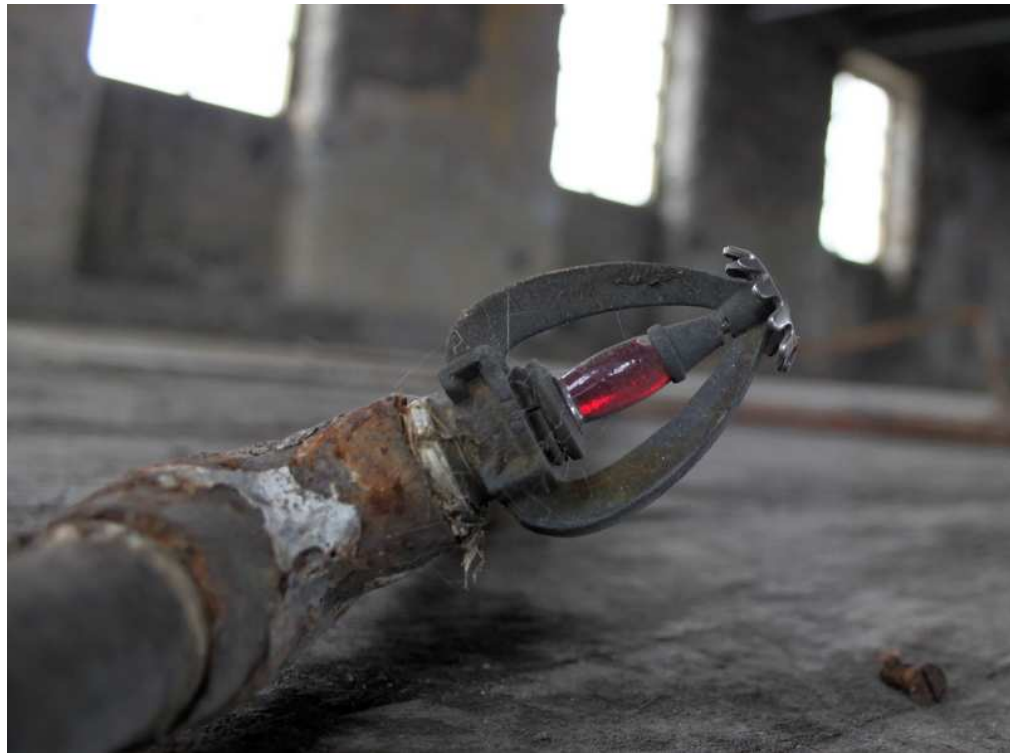
Plate 44: Glass sprinkler bulb
