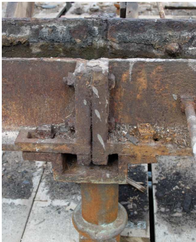
Plate 68: Jointing of valley gutter at column capital
