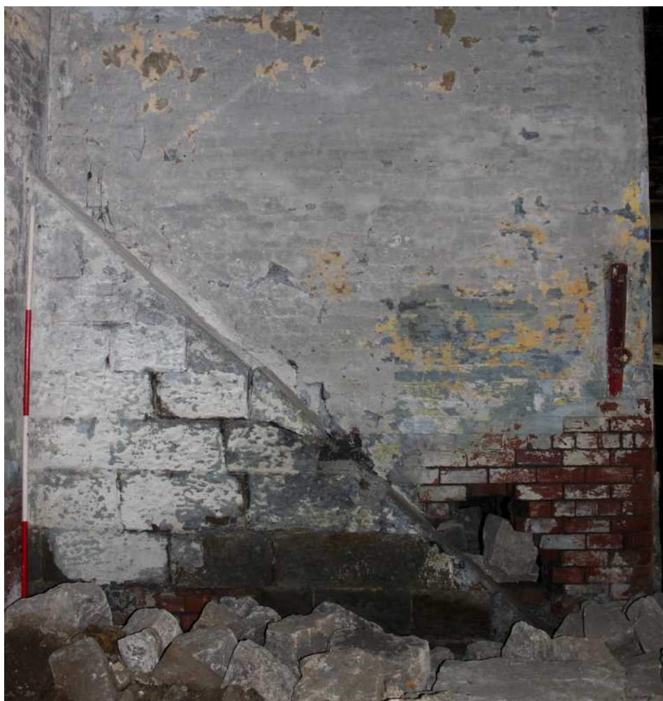
Plate 54: Reduced stone wall within later weaving shed, with blocked flue bottom left
