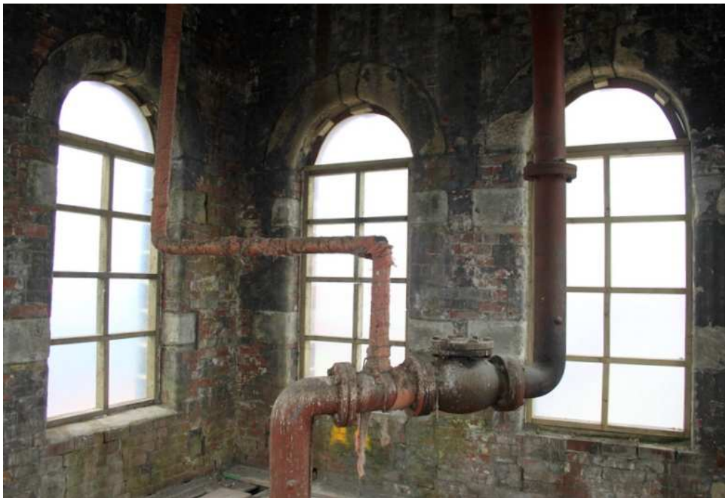
Plate 40: Round-headed windows in brick elevations on fifth floor of stair tower, with valve and spur on dog-legged main sprinkler pipe
