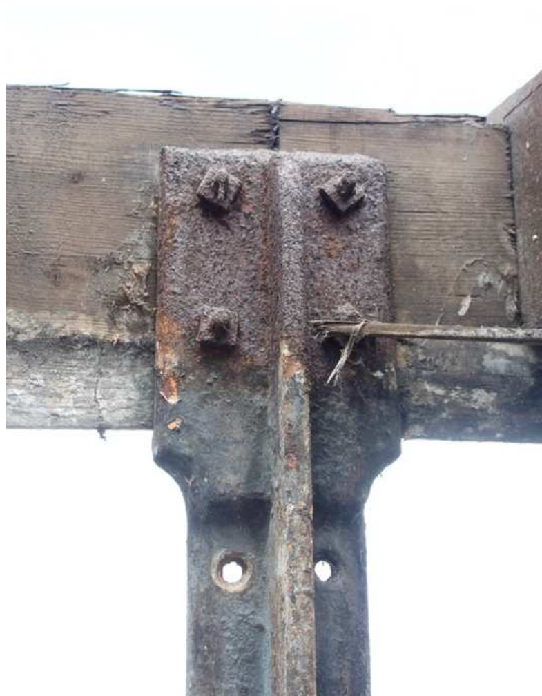
Plate 69: Head of cast-iron rafter in the weaving shed
