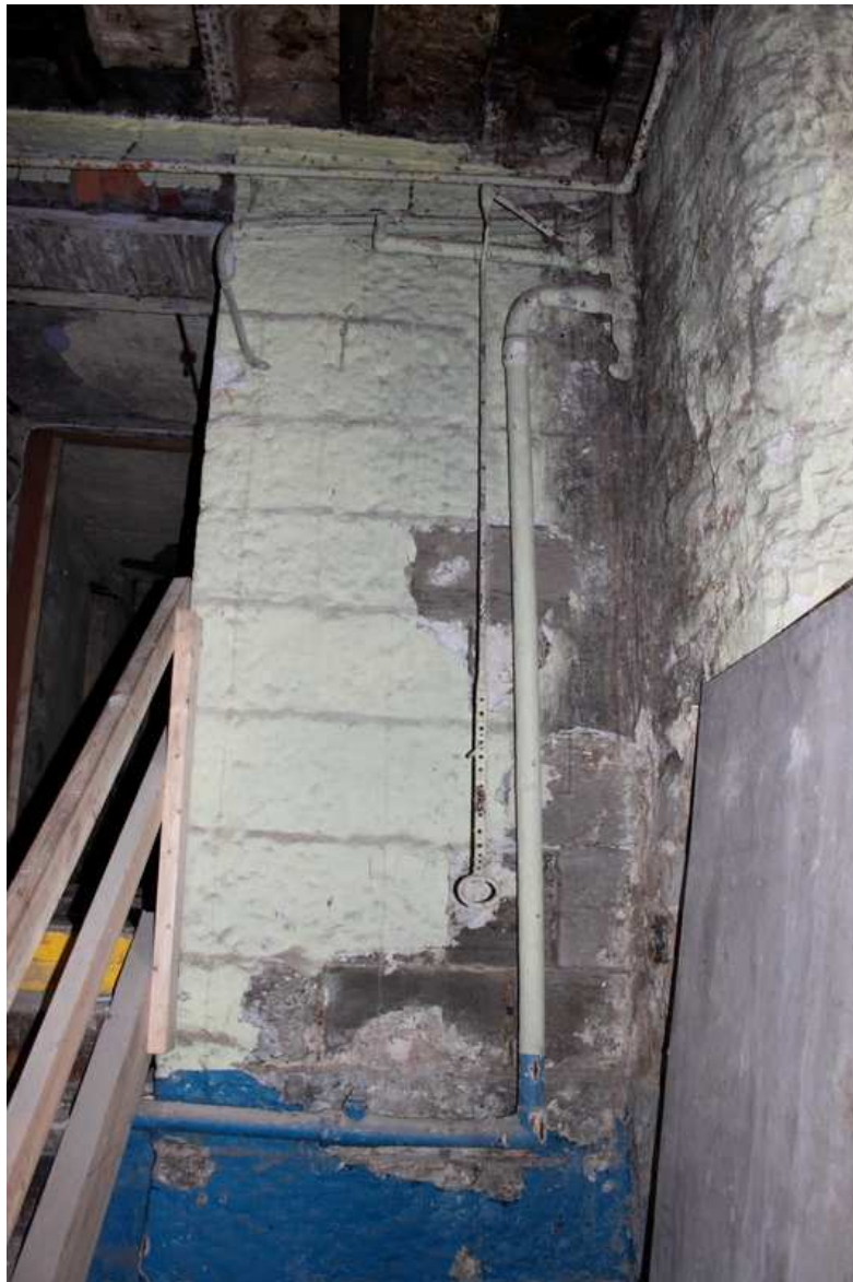
Plate 24: Control rod attached to water pipe at ground-floor level
