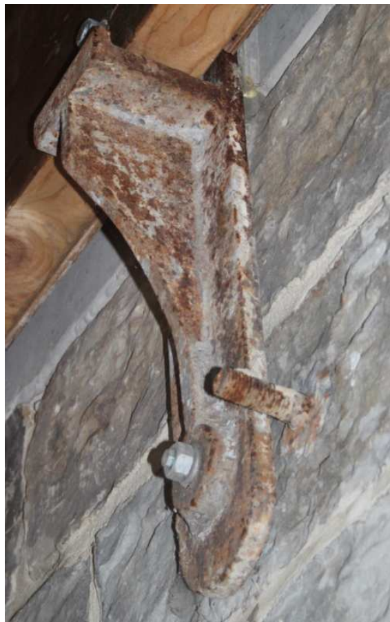
Plate 36: Corbel housing wall plate against south-east wall
