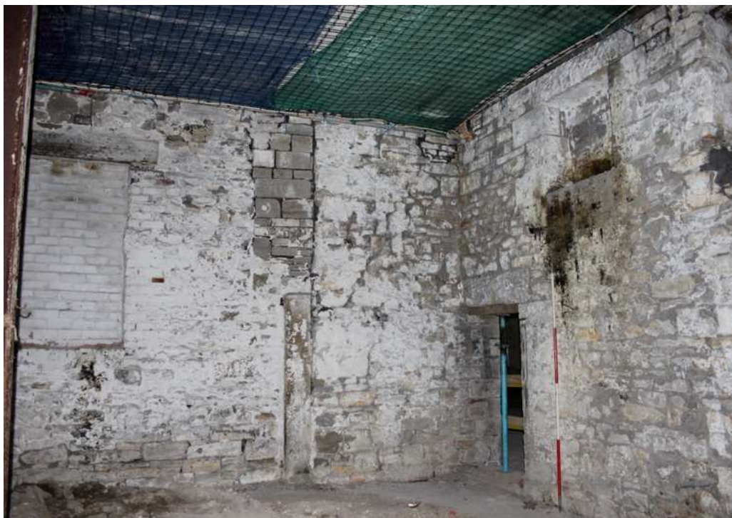
Plate 8: Southern corner of the engine house, showing scar of the original wall return, and bearing boxes in the extension
