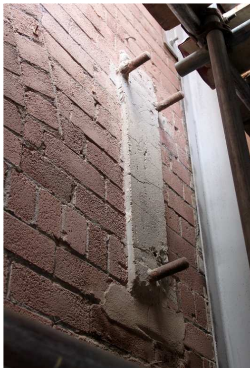
Plate 65: Bolting face for bevel gear in south-west wall of weaving shed
