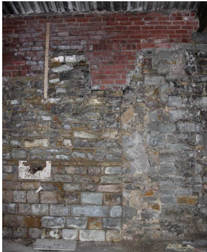
Plate 72: South internal elevation, showing butt joint in wall, and infilled bearing box
