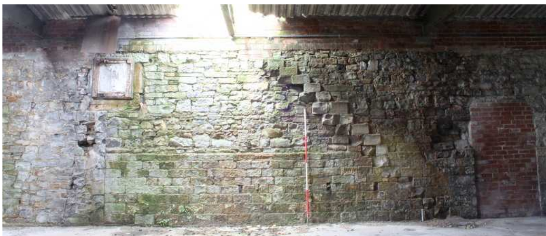
Plate 73: North internal elevation, showing butt joint in wall, extant bearing box, and removed stair
