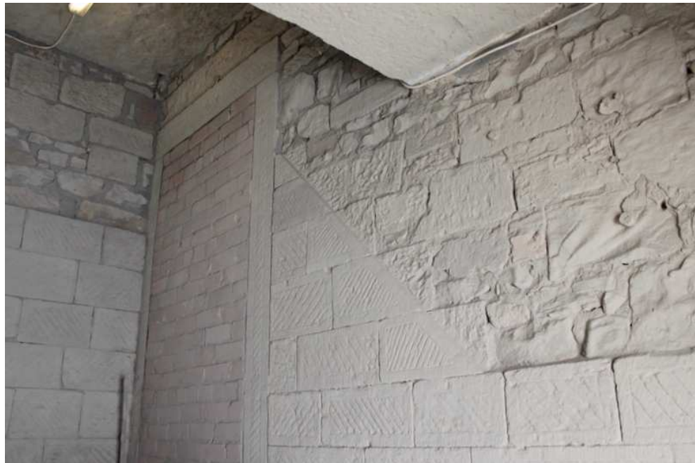
Plate 41: Decorative ashlar stonework below rubble construction within stair tower
