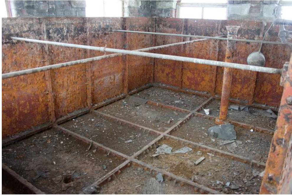
Plate 45: Construction of sprinkler system header tank
