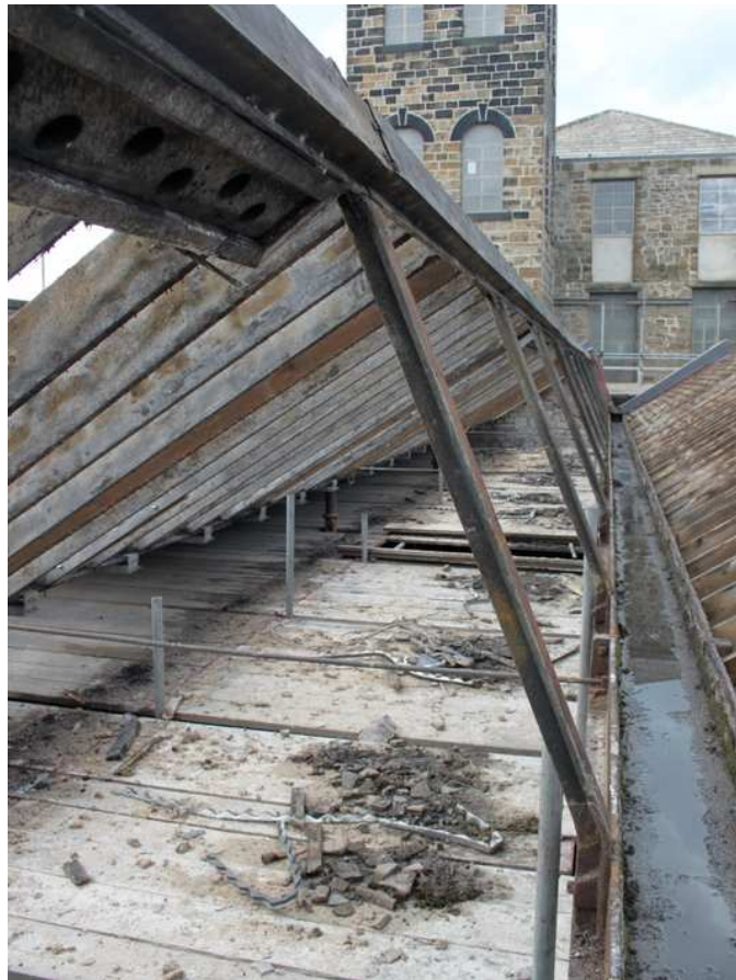
Plate 67: Detail of north-light roof construction
