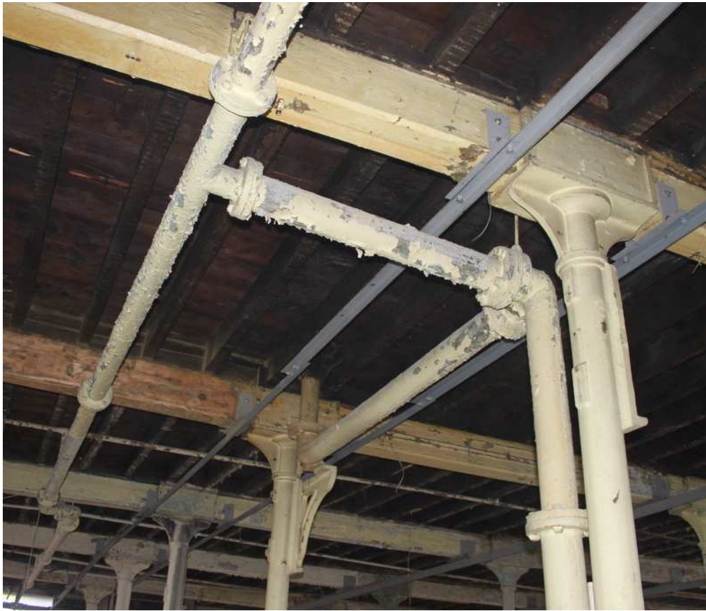
Plate 28: Detail of sprinkler system at first floor level
