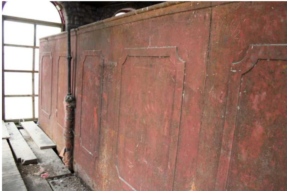
Plate 46: Decorative panelling of sprinkler system header tank
