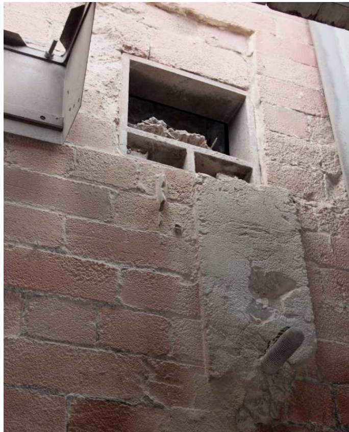
Plate 66: Bearing box above bevel gear in south-west wall of weaving shed
