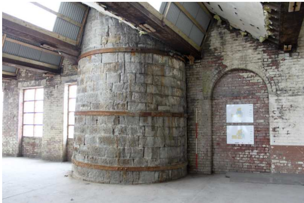
Plate 63: Chimney incorporated in weaving shed, with stub of line shaft hanger to right
