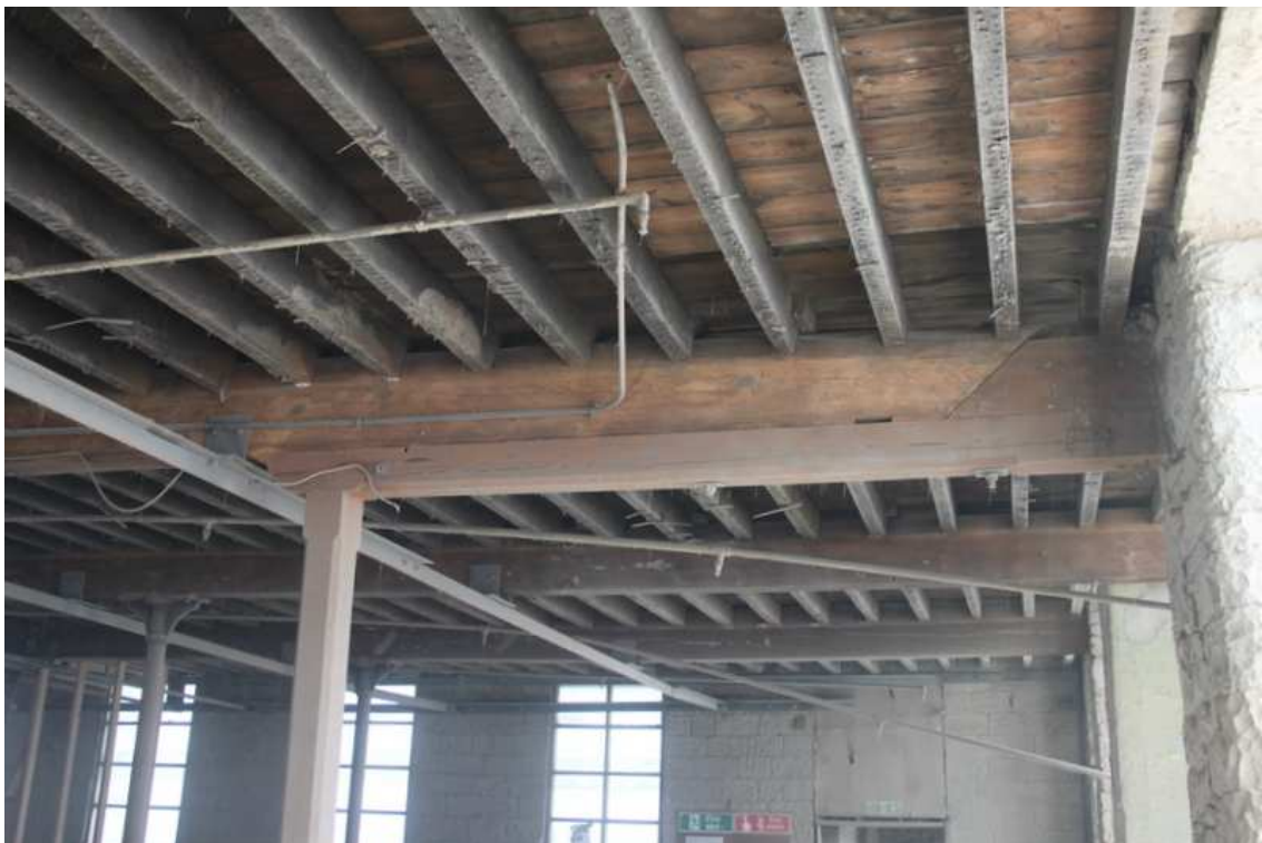
Plate 32: Spliced and propped beam at second-floor level
