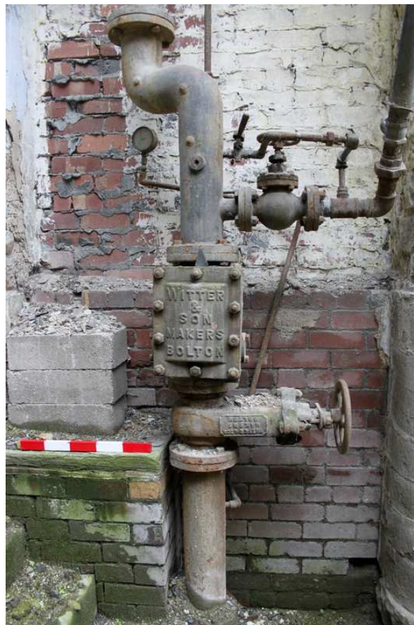
Plate 43: 'Christmas tree' valve of Witter automated sprinkler system
