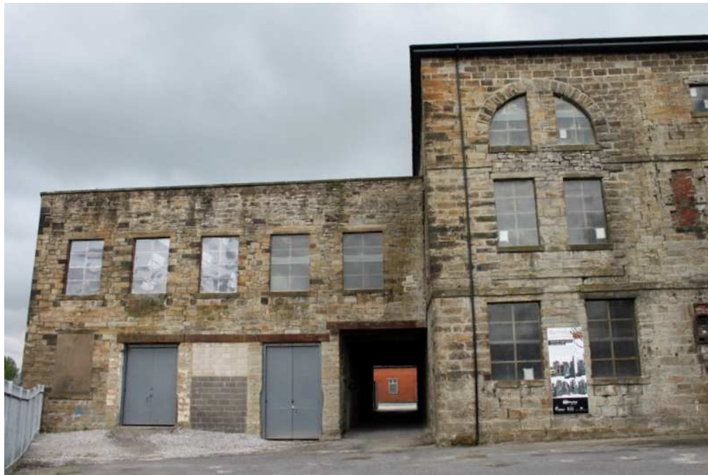
Plate 56: North-western face of preparation block / weaving shed, with enlarged doorway for insertion of Lancashire boiler
