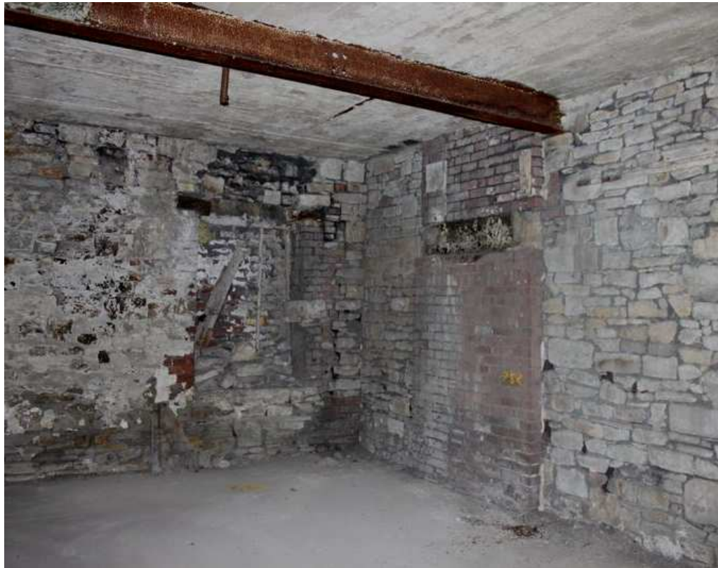
Plate 11: Blocked window, door and large bearing box, first floor, engine house
