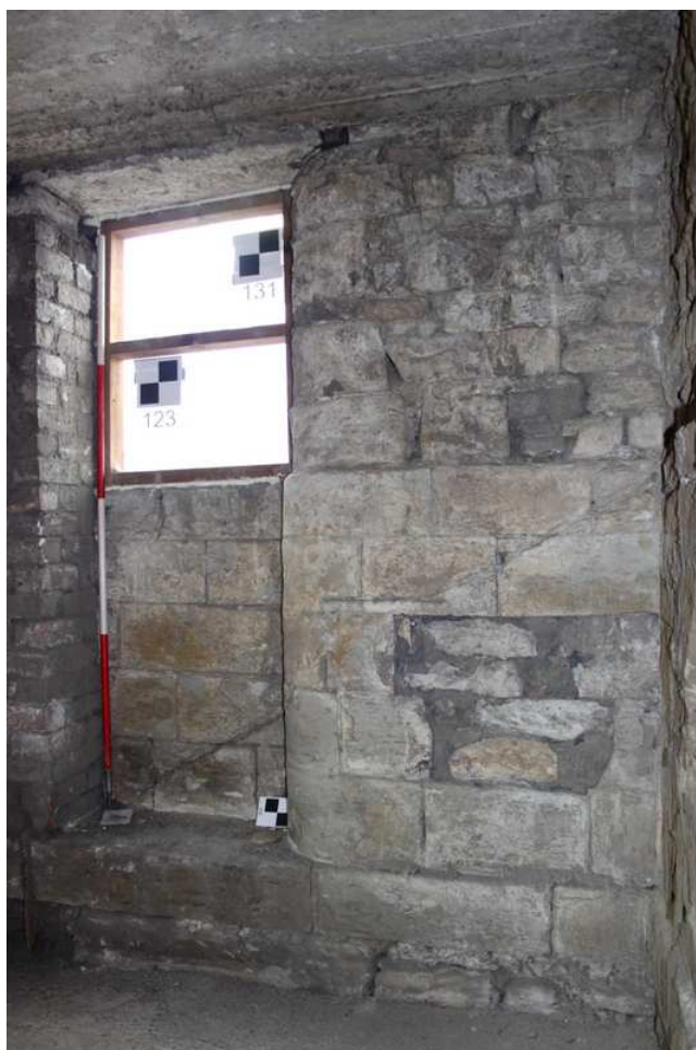
Plate 12: Scar of roof line within remodelled stairwell, engine house
