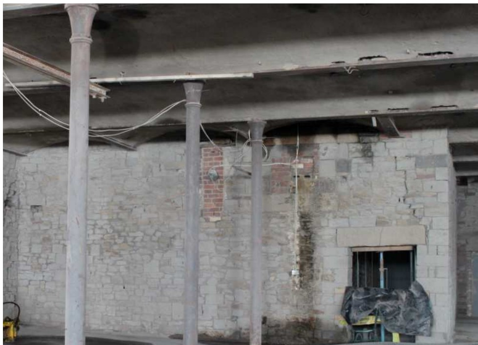
Plate 59: Vaulting alignments, scars for line shaft hangers, and blocked bearing boxes in engine house wall
