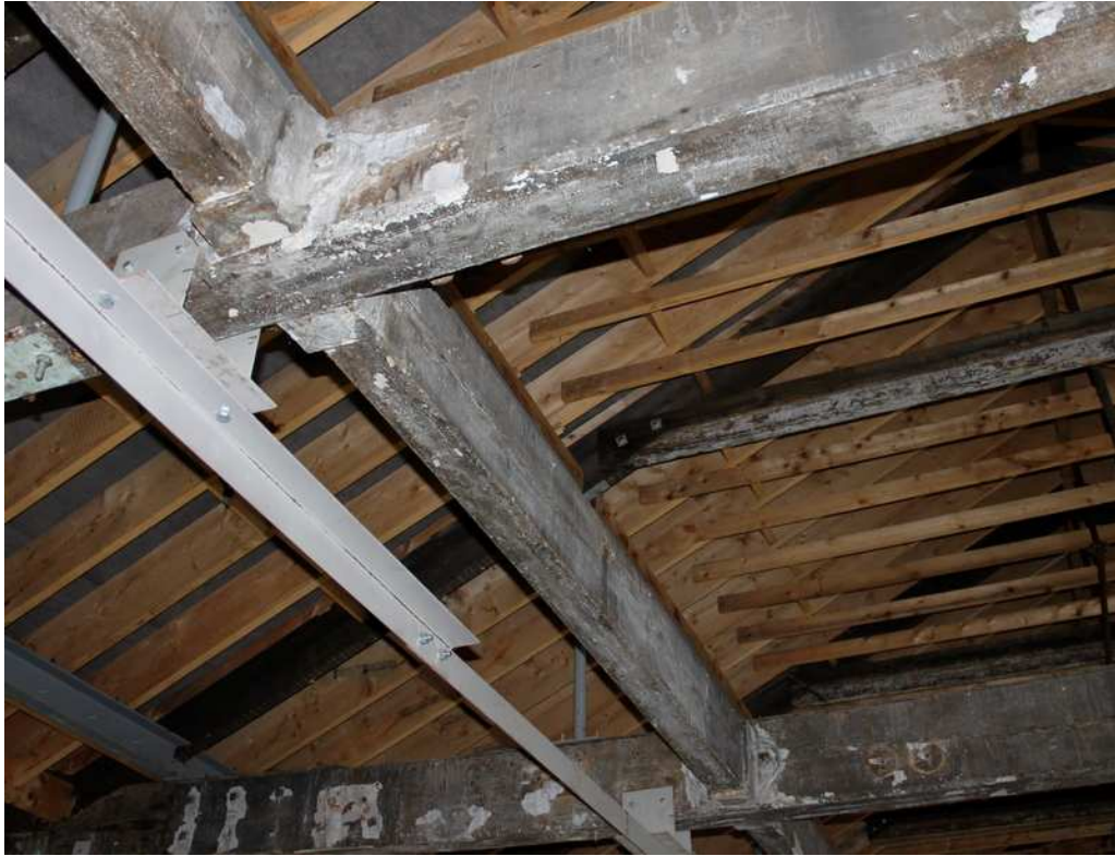
Plate 34: Trimmers between tie beams, housed in cast-iron brackets
