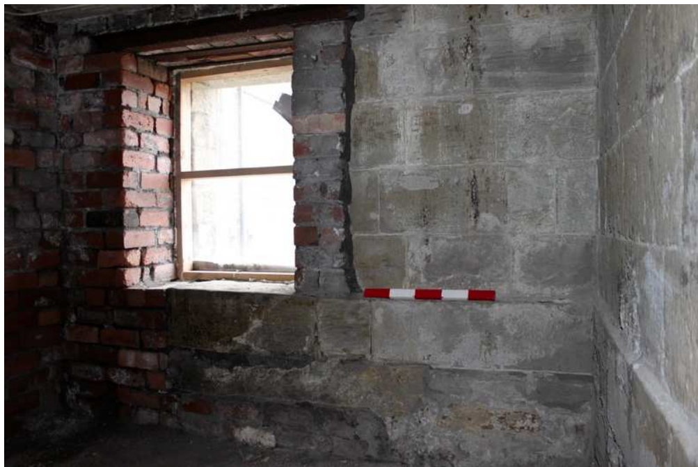
Plate 9: Extant elements of the original spinning block within the remodelled stairwell of the engine house
