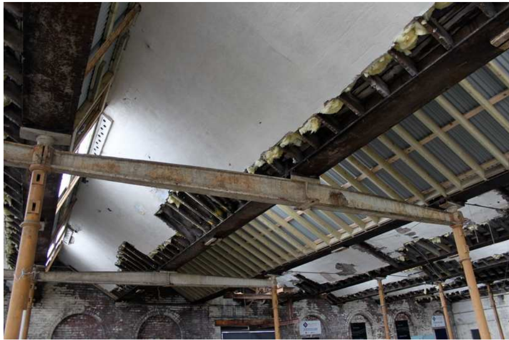
Plate 62: Whale-backed beams carrying roof valleys between column rows
