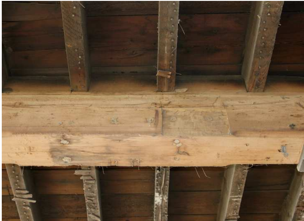
Plate 25: Stop-chamfers and bolt holes relating to original column position, first floor
