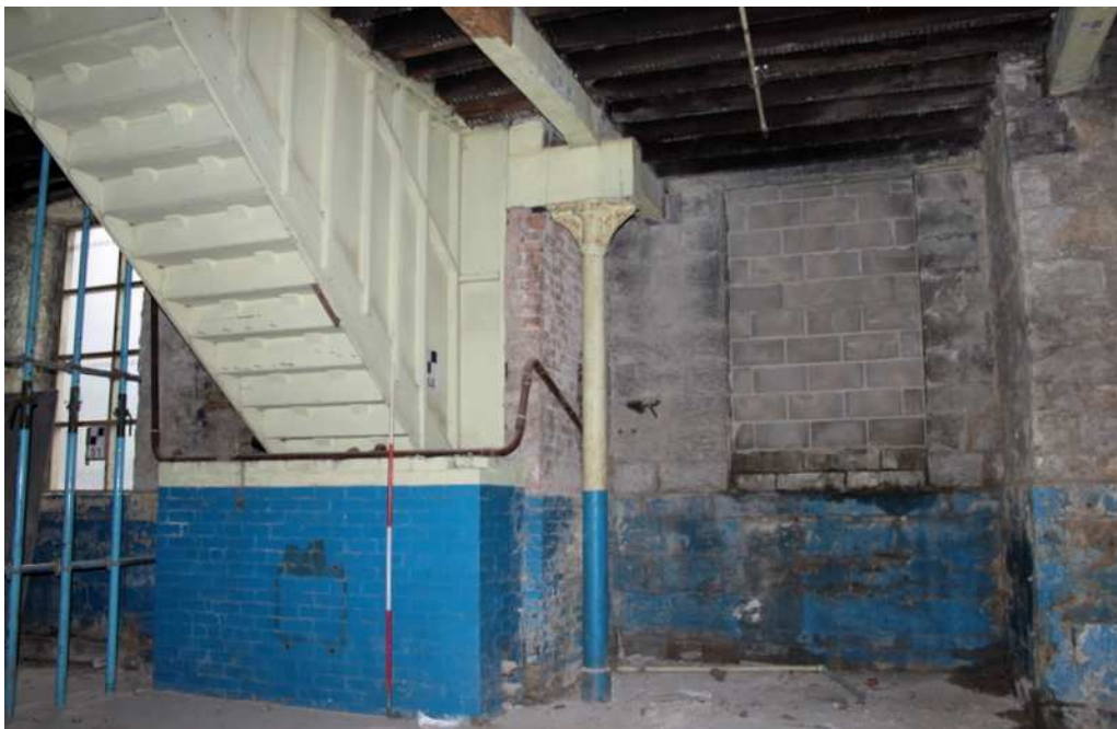
Plate 19: Projecting tower of south-west elevation with inserted stair and associated column
