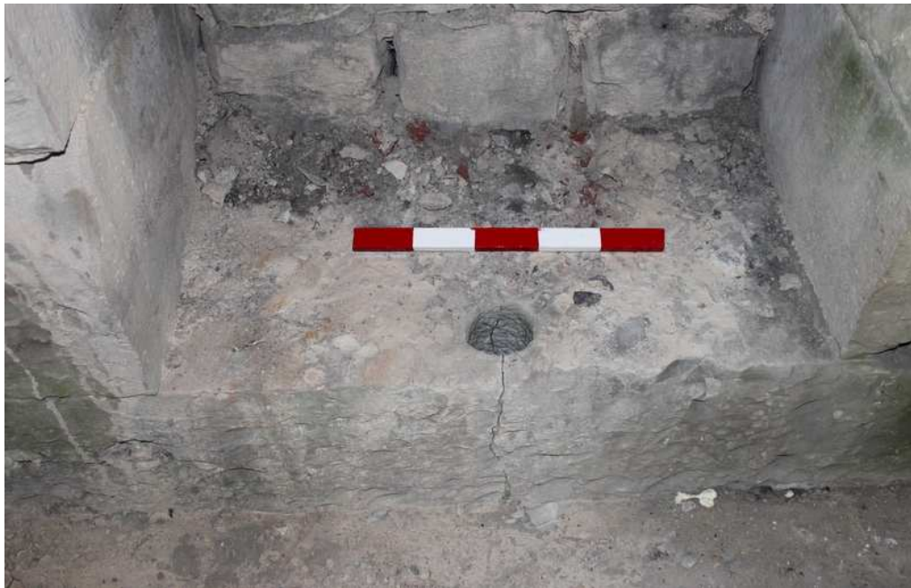
Plate 14: Detail of tying down bolt hole within second floor engine housing
