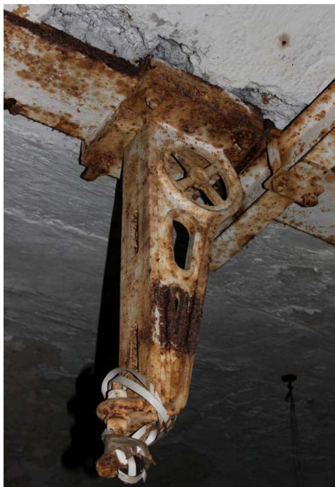
Plate 60: In-situ line shaft hanger in the weaving shed
